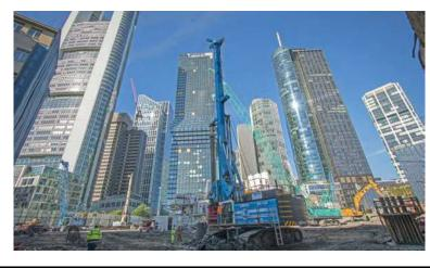
Due to space restrictions on the FOUR Frankfurt project, the buildings' basements are being built using the top-down construction method
